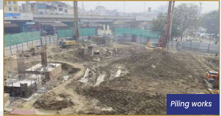
Column footing under progress
